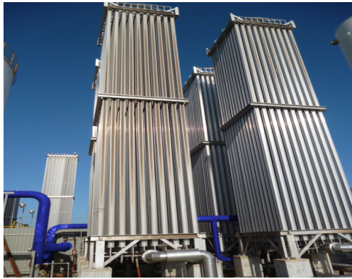
ATMOSPHERIC VAPORIZERS
