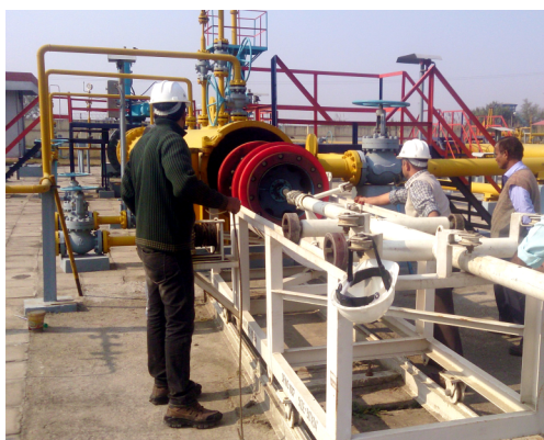
PIGGING PROJECT & PIG LAUNCHING STATION
